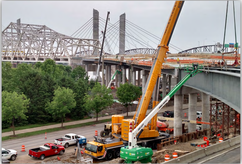
Sterett Crane setting bridge beams on the I-65/I-64 ramps.
