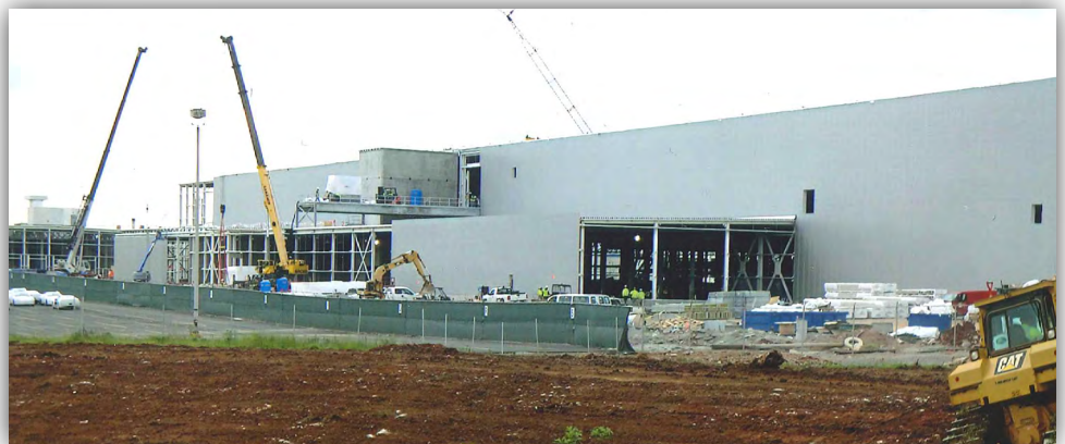
Paint Booth Expansion at the Corvette Plant in Bowling Green, KY
