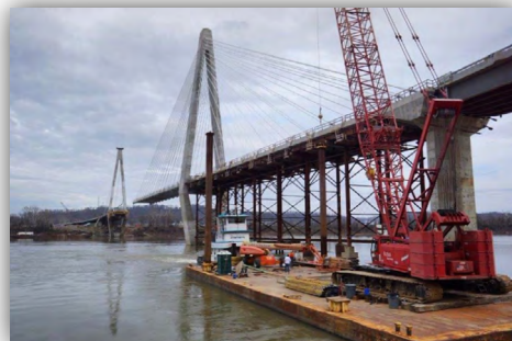
Ironton-Russell Bridge nearing completion that connects Ironton, Ohio with Russell, Kentucky.
